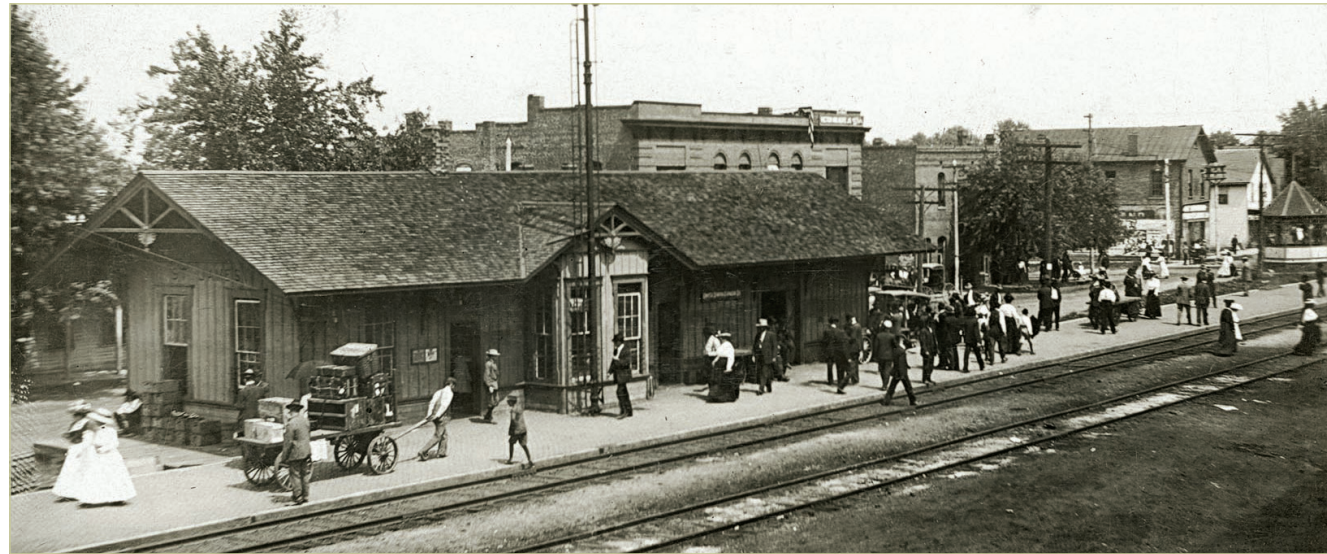
The Frisco Railroad depot at St. James, ca. 1910. The Phelps County passenger and freight depot is a classic example of structures common during the period.
